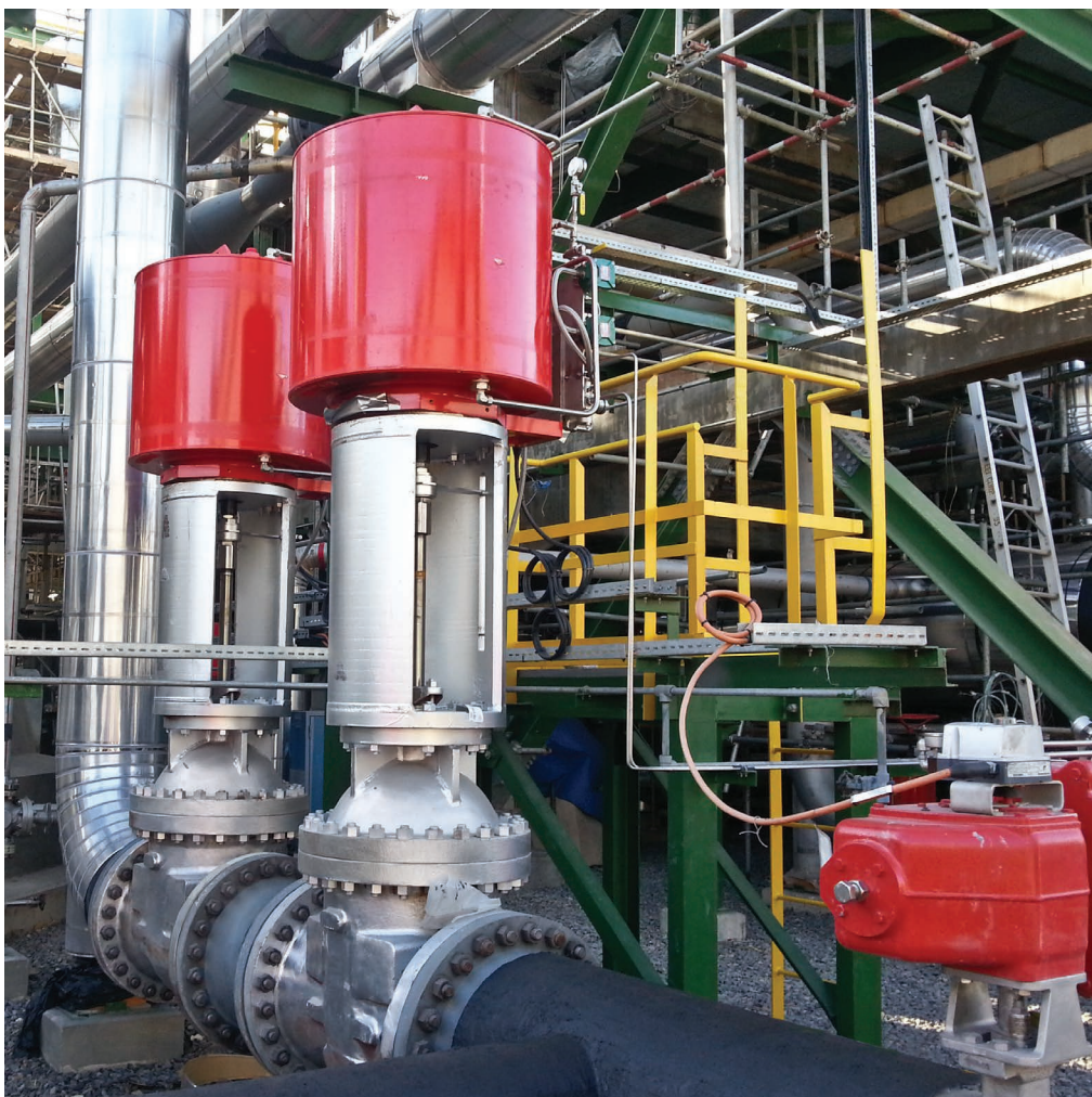
Two 18" Class 300 air-operated gate valve assemblies installed in the naphtha cracker plant
