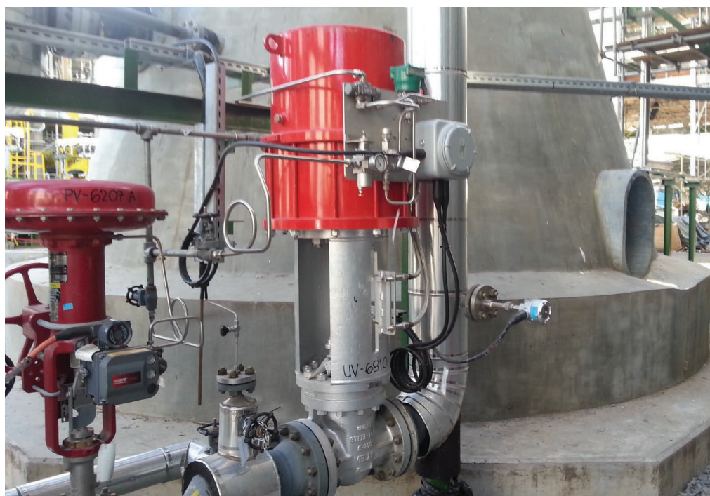
A 6" Class 300 air-operated gate valve assembly installed in the naphtha cracker plant
